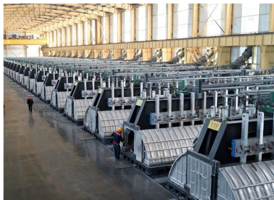
Figure 4. The potroom after the upgrade.
