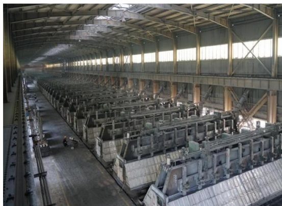
Figure 3. The potroom before the upgrade.
